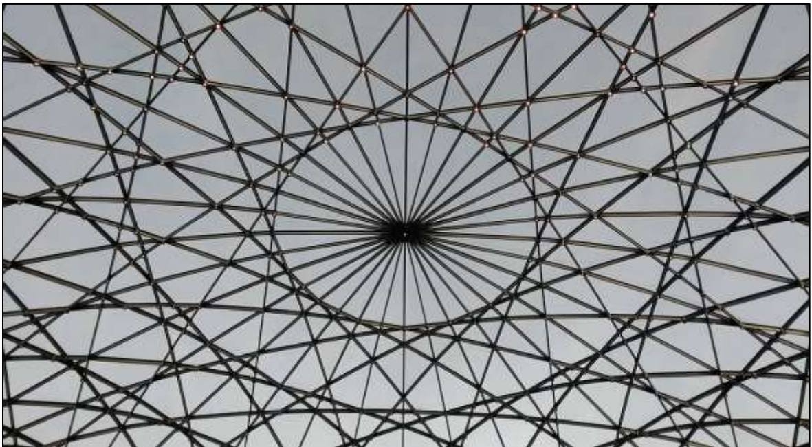
Fig. 1-1 The grid roof of the National Maritime Museum in the Netherlands (Pascal, 2021).
