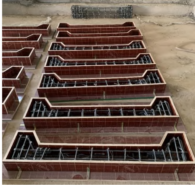
Figure 3.12: Placement of steel cages within formworks
