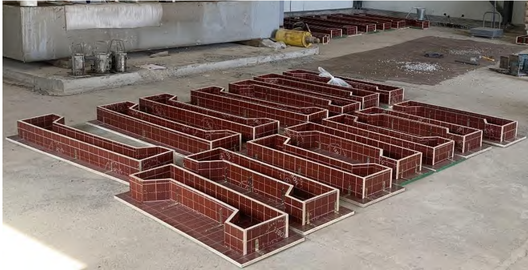
Figure 3.11: Column formworks for casting concrete
