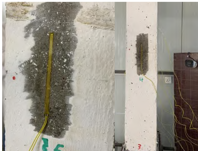
Figure 3.20: Concrete strain gauge installed on the column.
