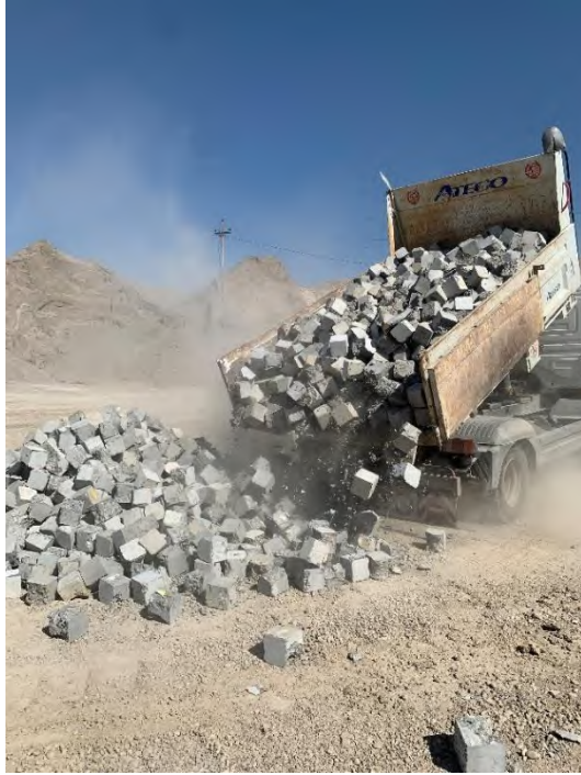
(a) Collecting waste concrete
