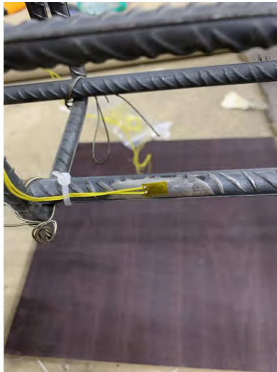
Figure 3.21: Steel strain gauge installed on tension and compression faces bars.
