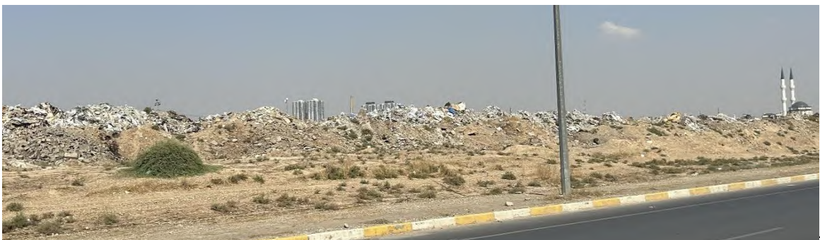
Figure 1.1 Construction and demolition waste disposal in a landfill (Erbil).
