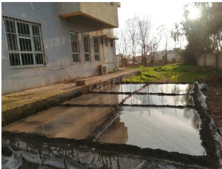
Fig. 3- 9 Curing of the concrete
