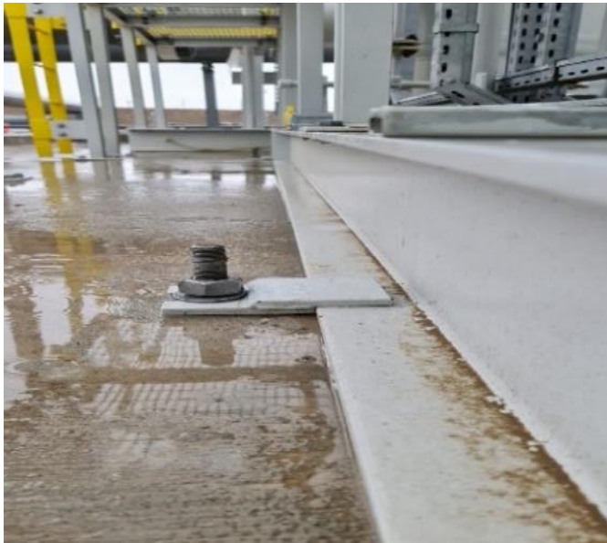
Fig. 1- 2 KAR company equipment Fixing on RC Floors,2020
