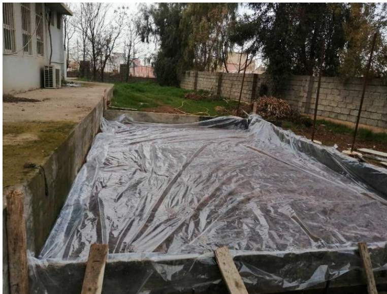
Fig. 3- 7 Site preparation for the concrete slab
