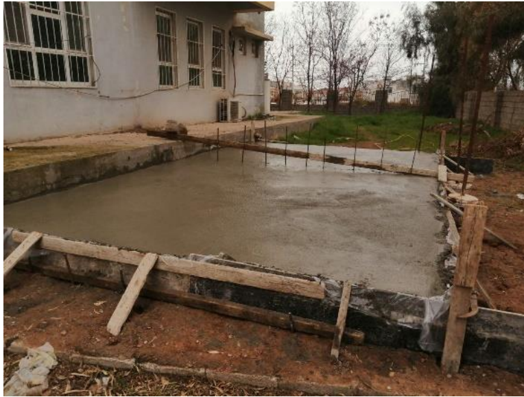
Fig. 3- 8 Placement of the concrete
