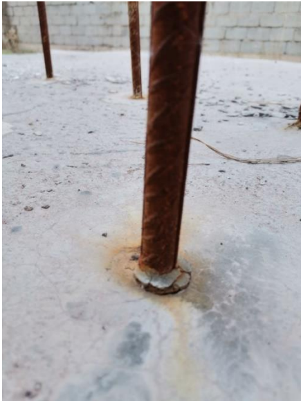
A) Concrete -grout interface (Mode 3)
