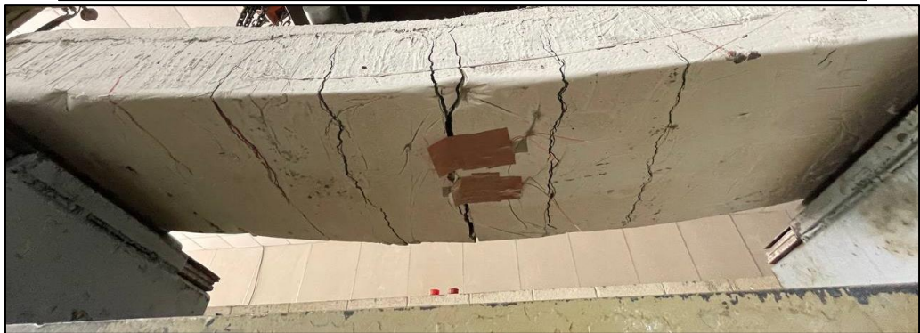
Figure 4.28: VG mold Crack pattern
