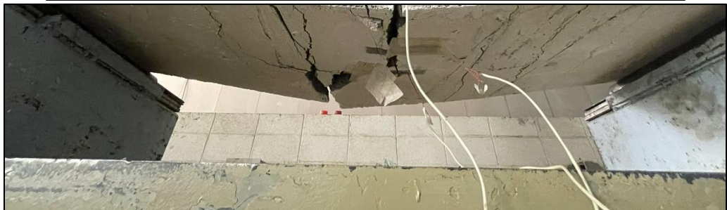
Figure 4.26: R-UHPC15 mold Crack pattern
