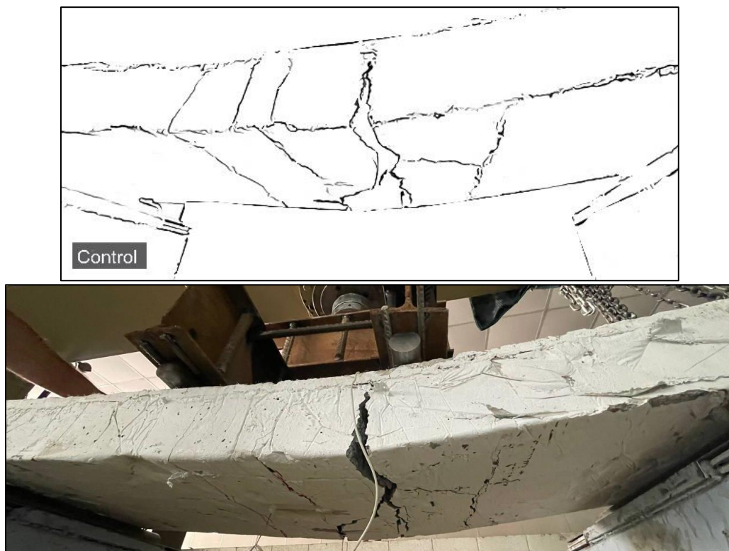
Figure 4.20: Control mold Crack pattern
