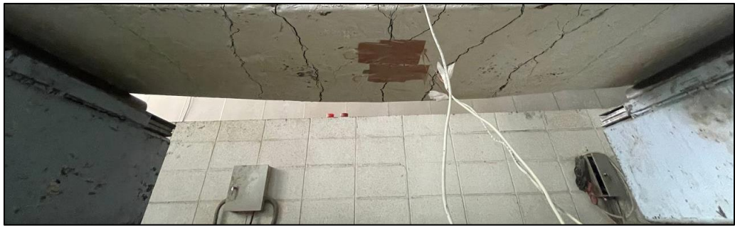
Figure 4.25: R-UHPC10 mold Crack pattern
