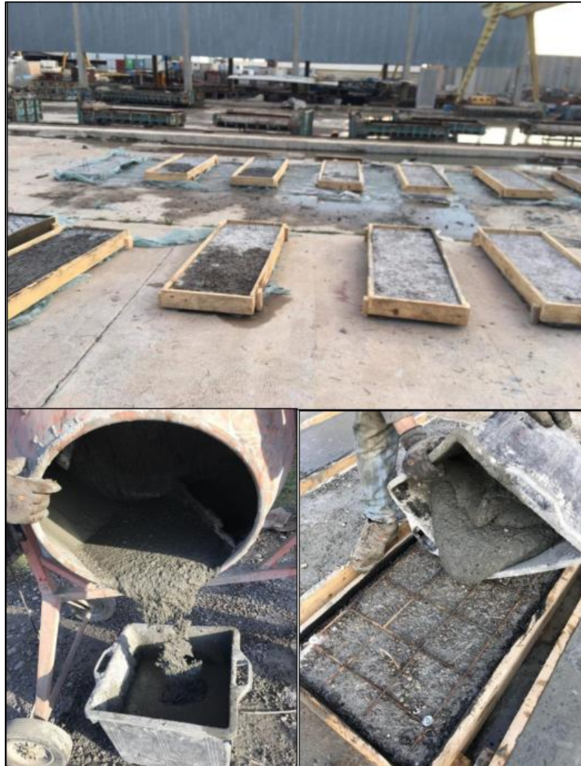
Figure 3.11: Casting overlay concrete
