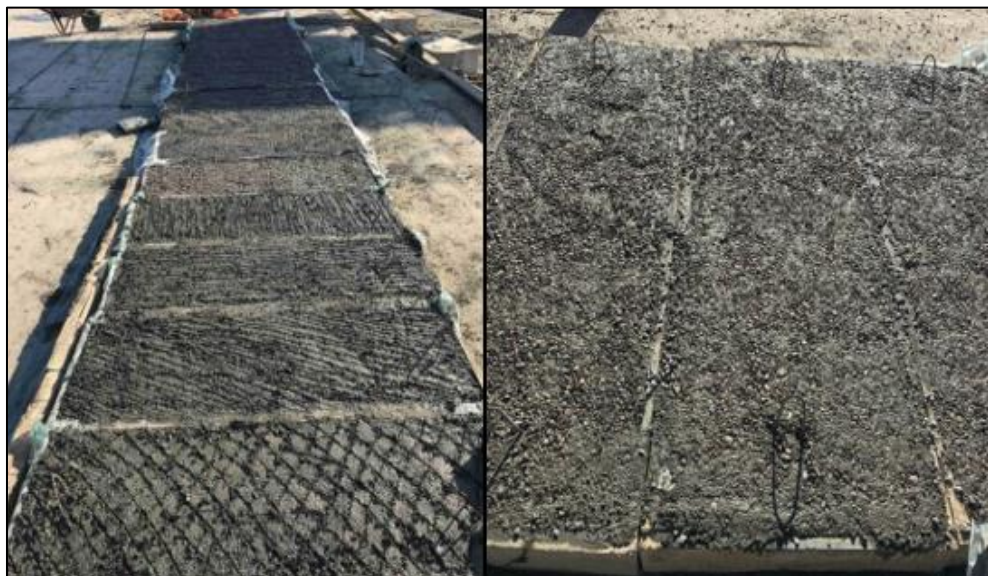
Figure 3.10: Casting substrate concrete
