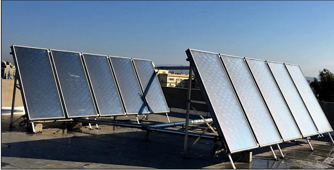
Figure 4.4 Photograph of the FPSC.
